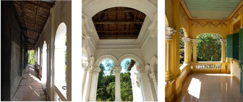
Figure 3. Shading and rain protection solutions with sloping roof and porch in the house of Mr. Xoat (left, middle) and Mr. Ba Duc (right).
