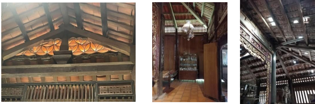
Figure 5. Natural lighting solution with gable roof and slatted wall in Mr. Kiet's house.
