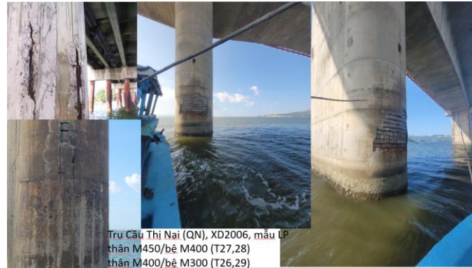
Figure 2. Corrosion of reinforced concrete in a Marine Environment after 20 years of Construction.
