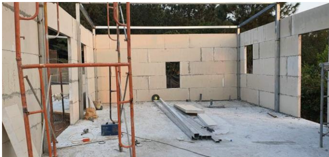
Figure 9. Precast house constructed with lightweight concrete [31].
