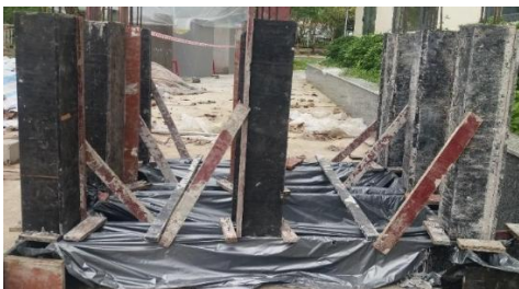
Figure 7. Installation of formwork and reinforcement and casting of concrete columns.
