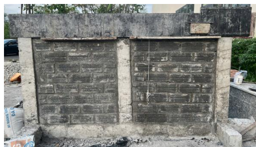
Figure 11. Frame after casting the upper beam.
