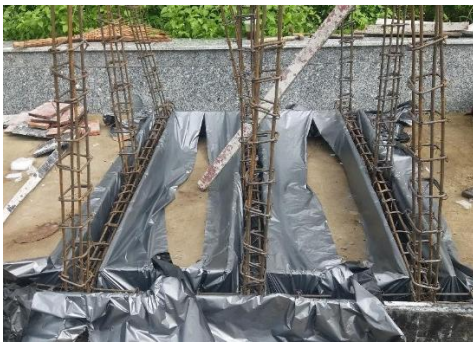
Figure 6. Installation of formwork and reinforcement for the base beam and columns.
