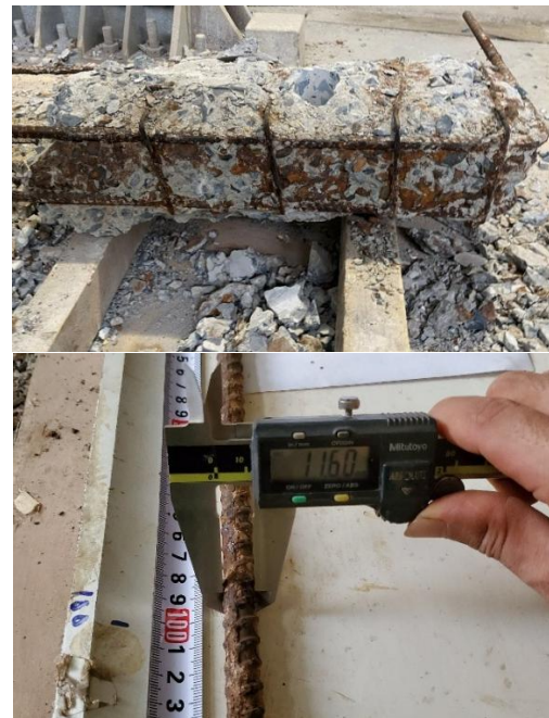
Figure 2. Survey of steel reinforcement diameters.
