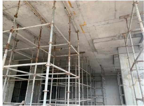
Figure 1. Third-level reshoring after removal of mushroom slab formwork.
