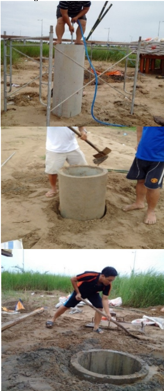
Figure 6. The process of installing well pipes.
