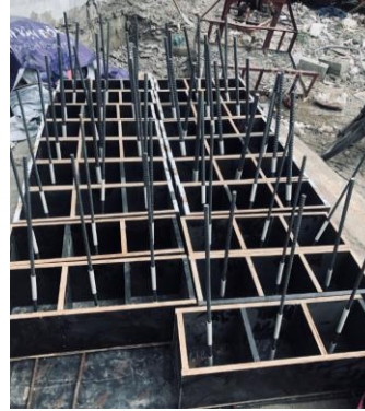
Figure 7. Set up steel bars.
