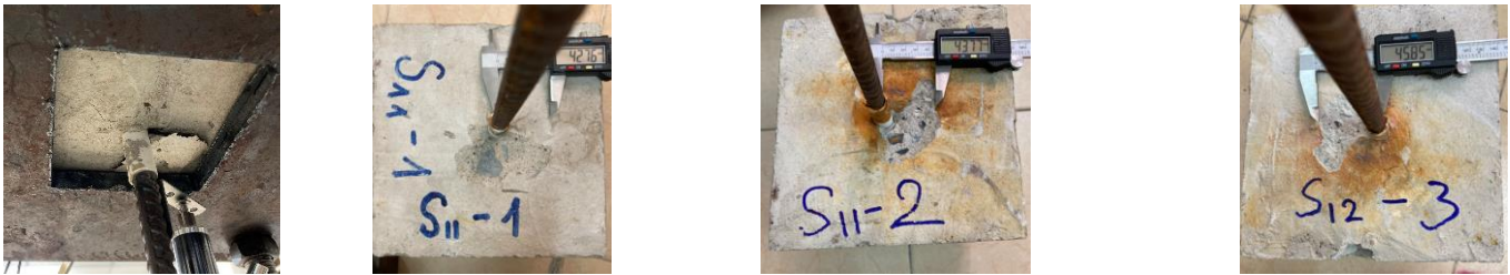
Figure 18. Corrosion-induced cracks of reinforcement D12.
