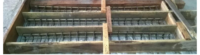
a) Reinforcing cages located in the wooden form
