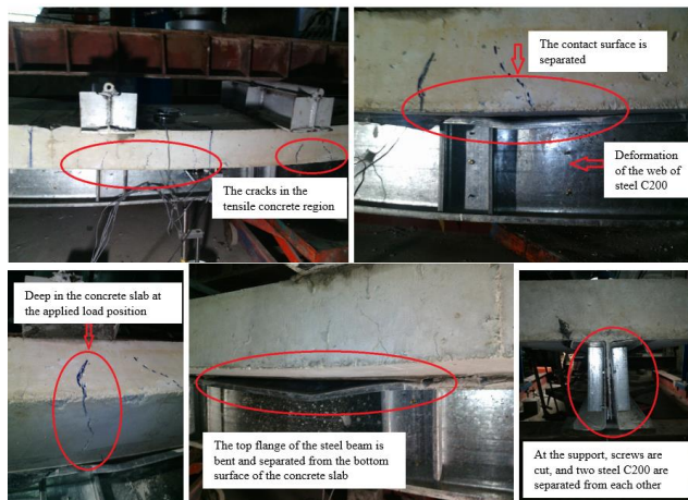
Figure 13. The failure mode of Beam 2.
