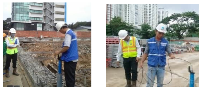
Figure 3. Monitoring the Wall Deformation [16].
