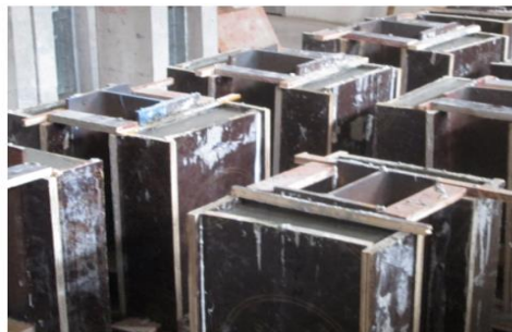
d. Specimens after concreting
