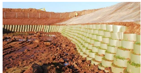
Figure 7. Structure of reinforced gravity retaining wall using Neoweb material.
