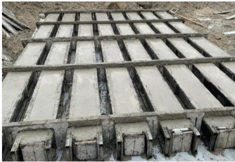
a. Concrete piling casting
