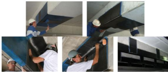
Figure 2. Construction steps for FRP fiber bonding to reinforce reinforced concrete structures [6, 7].
