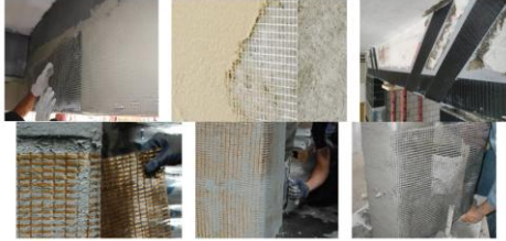
Figure 3. Construction of FRP fiber bonding to reinforce reinforced concrete structures [8, 9].
