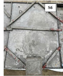
d) pouring of concrete (S6)
