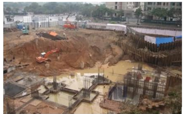
Figure 1. Occurrence of muddy water entering the base of the foundation pit.
