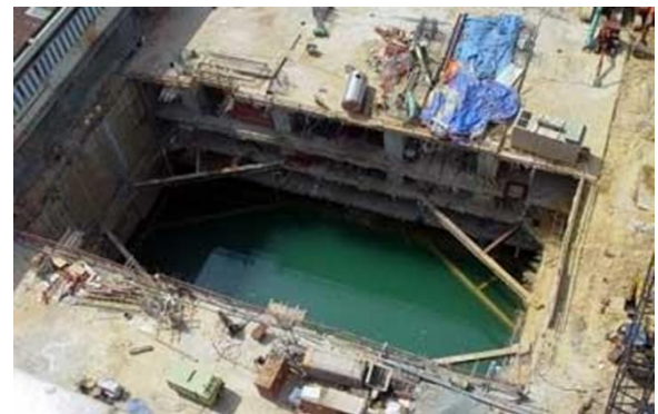
Figure 2. Water carries soil and sand into the basement.
