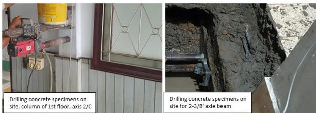
Figure 2. Drilling concrete specimens at the site.
