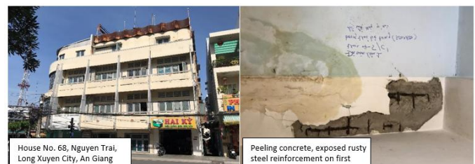
Figure 1. Survey recorded concrete cracking and steel rusting.
