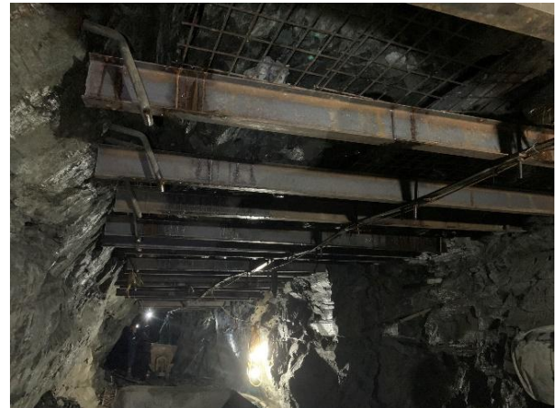
Figure 9. Some images of mine tunnel support using steel bolt-beam structures.
